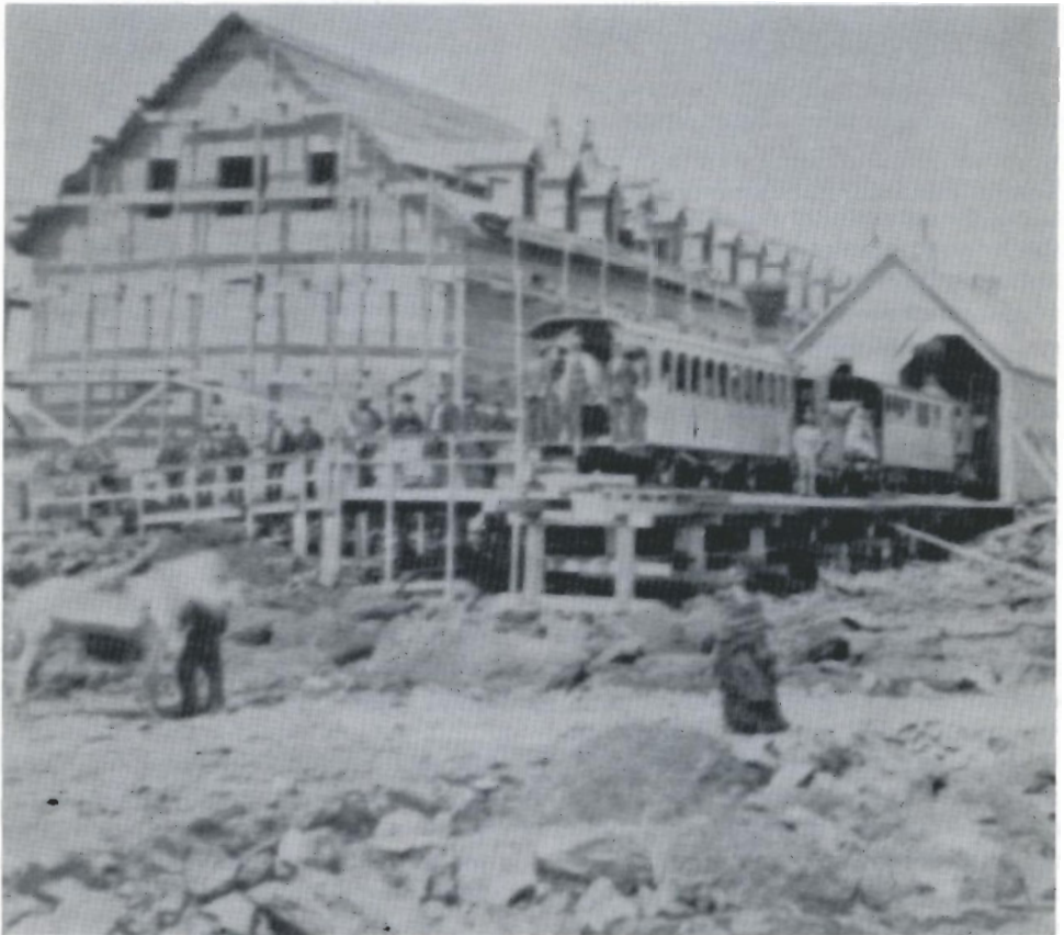
New Summit House under construction, 1873.
