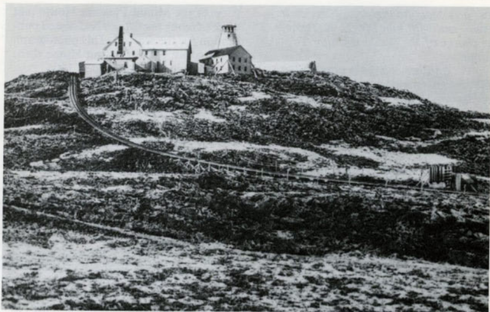
The Summit Colony from the northeast. Left to right: the kitchen sheds, the gable end of the main building, the ell built in 1874, the annex built in 1884, the U.S. Coast and Geodetic Survey tower, and Tip-Top House. [New Hampshire Historical Society]
