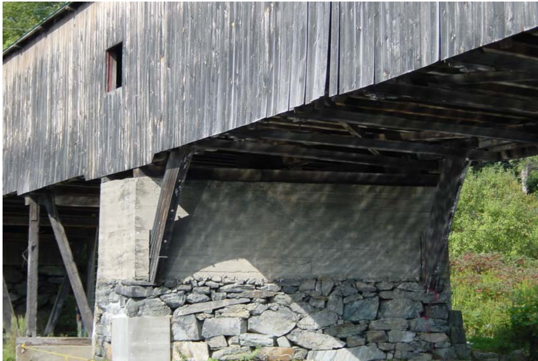
East face of Pier 3, Bath Village Bridge
