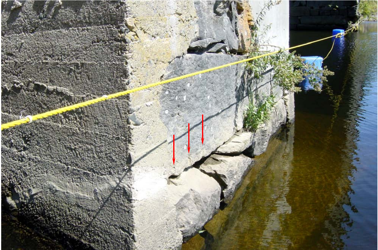
South face of Pier 3, Bath Village Bridge
